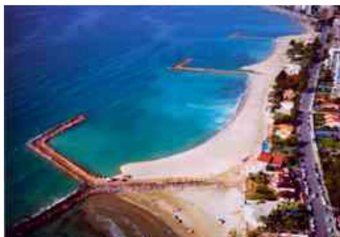
The purpose of the project was to create a stable beach for the use and enjoyment of the public, both local and from other areas. This required building two new central breakwaters of riprap and extending the two breakwaters at the ends, as well as providing 300,000 m<sup>3</sup> of gravel to regenerate the beach. The beach was also provided with a pinewood pedestrian walkway to connect to the two adjacent beaches, as well as services of lighting, showers, etc.
