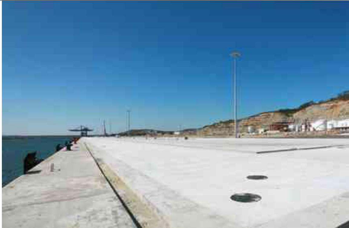
Independent drainage was also built for the future bulk solids and loading area. This drainage was built with a GRP sewer 1000 mm in diameter and discharges into a containment pool from which the water is pumped for treatment in treatment plants.
