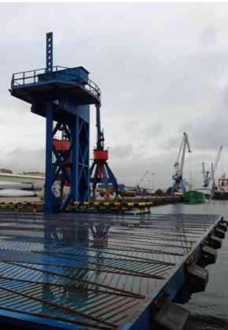
The works under this project are located at the end of the dock, where the North and Fernández Ladreda closing piers meet. There the foundations are at -6 (where Fernández Ladreda pier is grounded) and -10, the latter results from the dredging done to recently build the North pier.
