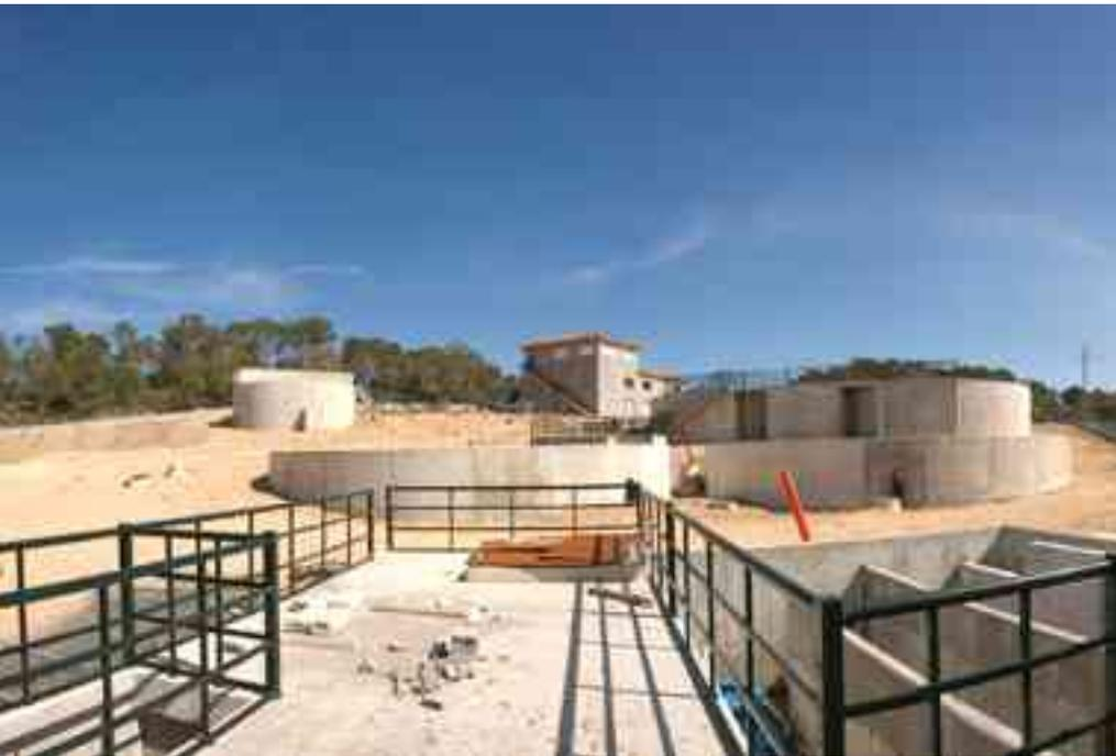
The purpose of the project was the building of the waste water treatment plant in Cala Tarida (Ibiza), to concentrate the treatment of sewage from this tourist area in a single installation. To guarantee the proper functioning of the installations it was necessary to consider the important seasonal variation of the population, that greatly affects the choice of treatment process given the inertia of the biological processes under wide variations of load and flow.
