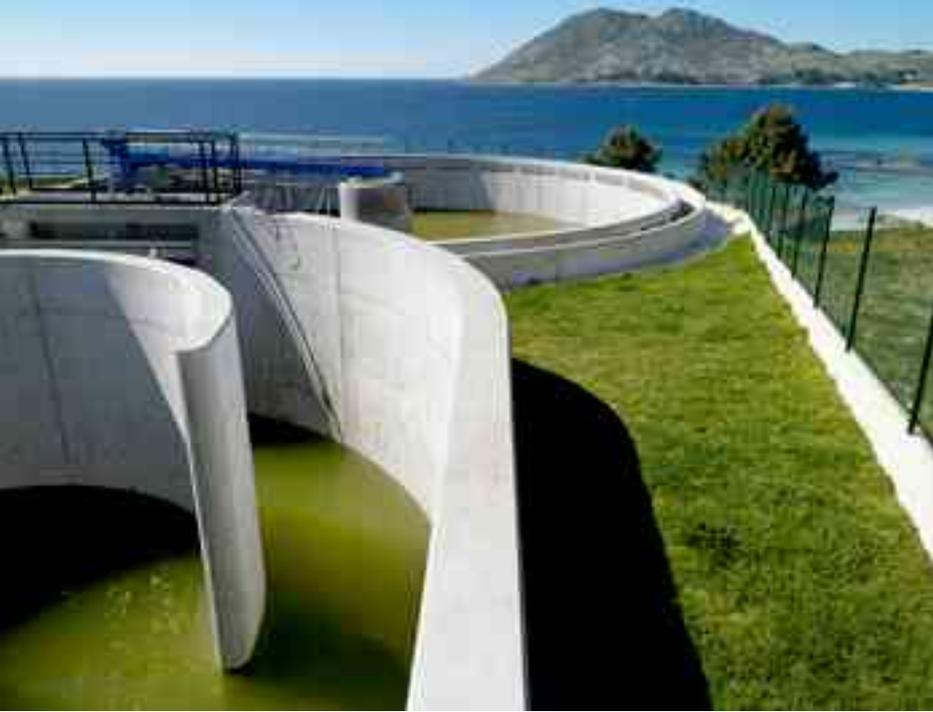
The purpose of this project was to collect sewage generated in Muros for its treatment and discharge to the sea via an underwater outfall, for which three pumping stations were built, designed with attached storm tanks and pumping as well as the building of various gravity sewers.
