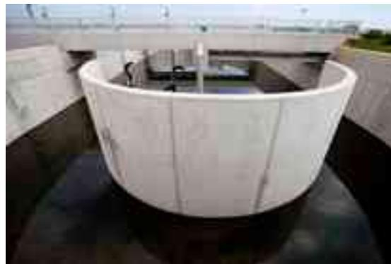
The WWTP is based on an activated sludge system at very low load, that is, with prolonged aeration using a carousel with two channels. It also has new covered pre-treatment, a new secondary clarifier, deodorising by bio filter as well as new physical and chemical treatment in case the biological treatment is put out of service by an emergency.
