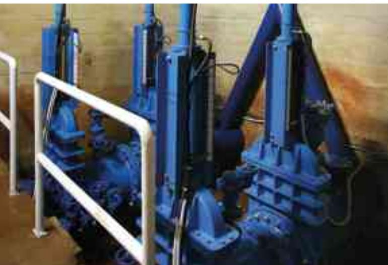
The work undertaken mainly consisted of rehabilitating the control room, replacing the bottom outlets and the intake, installing a hydraulic set for operating them as well as a new gantry crane for installing and handling the valves.
