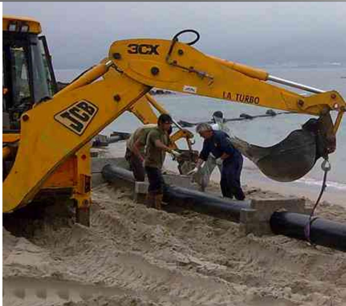
It is 1,200 ml long. It was built with PEAD piping of 200 mm diameter and discharges at -21 ml. A total of 402 concrete ballast units were used for anchoring it and 138 for fixing it to the sea bottom. The cost for developing this channel amounted to EUR 124,935.
