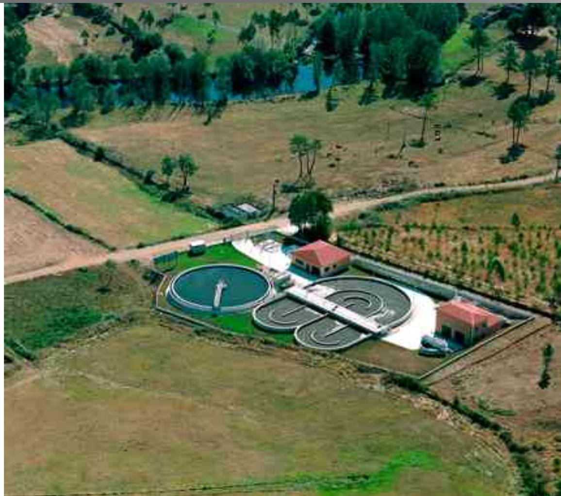
The WWTP it is based on a biological process in a carousel type line with stirring systems and prolonged aeration with activated sludge.
