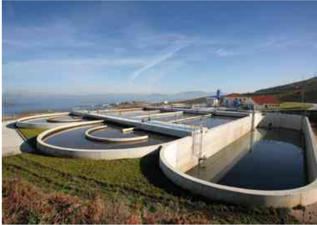
Treatment is of the activated sludge biological type or by prolonged aeration with two carousel reactors aerated by surface rotors, a prior storm tank and secondary clarifying. Drying by centrifuge.
