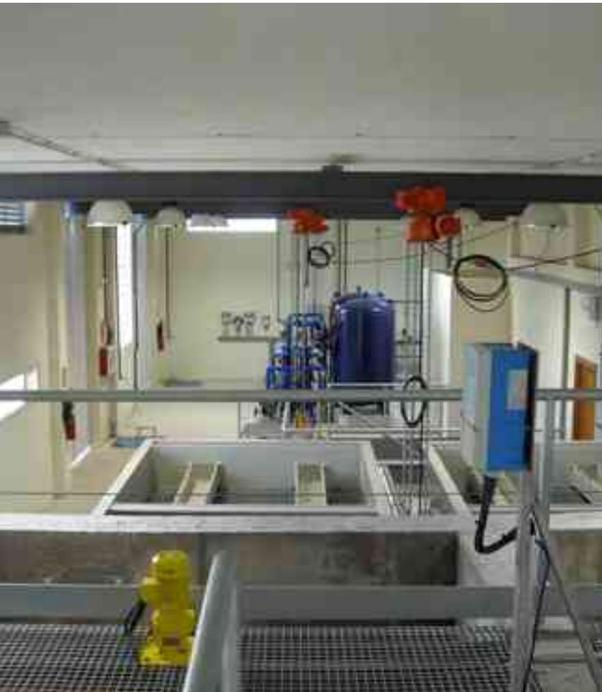
The water enters the quick mixing chamber (2.08 m<sup>3</sup>) where sodium hypochlorite and aluminium hydrochloride are added before it passes to two independent chambers each of 7.80 m<sup>3</sup> where coagulation and flocculation take place to favour clarifying. Clarifying takes place in two low speed ascending lamellar clarifiers with an area of 52 m<sup>2</sup> in two independent lines.
