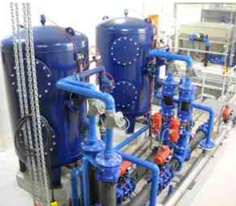
After the exit from the filters, post-chlorination takes place using sodium hypochlorite.
