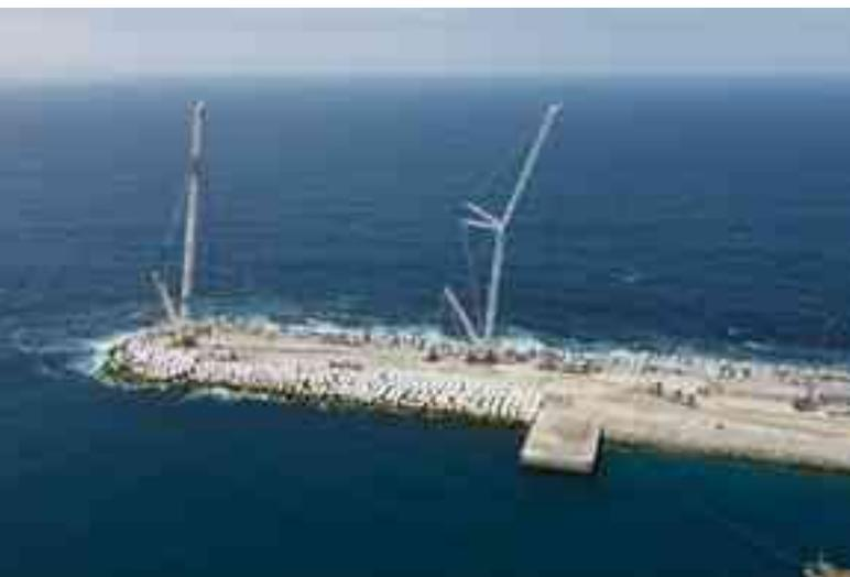
A transverse mole of precast concrete caissons (51.10 x 20.50 m) with a depth varying from 21 to 27 m long. An edge beam 5.35 m deep is located on the caissons to support the outer rail of the crane, the mooring bollards and the fenders. The crane's inner track is 18 m from the outer one on a 1 m beam with a concrete slab 45 cm thick between the two rails.
