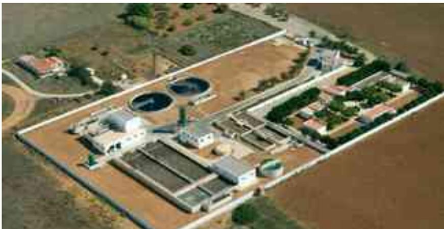
The WWTP is based on an activated sludge system with A/O/A/O type nitrification and denitrification. It also has new pre-treatment and a covered tank for receiving the contents of cesspits, sludge thickener, two new secondary clarifiers, as well as physical and chemical treatment with lamellar clarifying in case the biological treatment is put out of service by an emergency.
