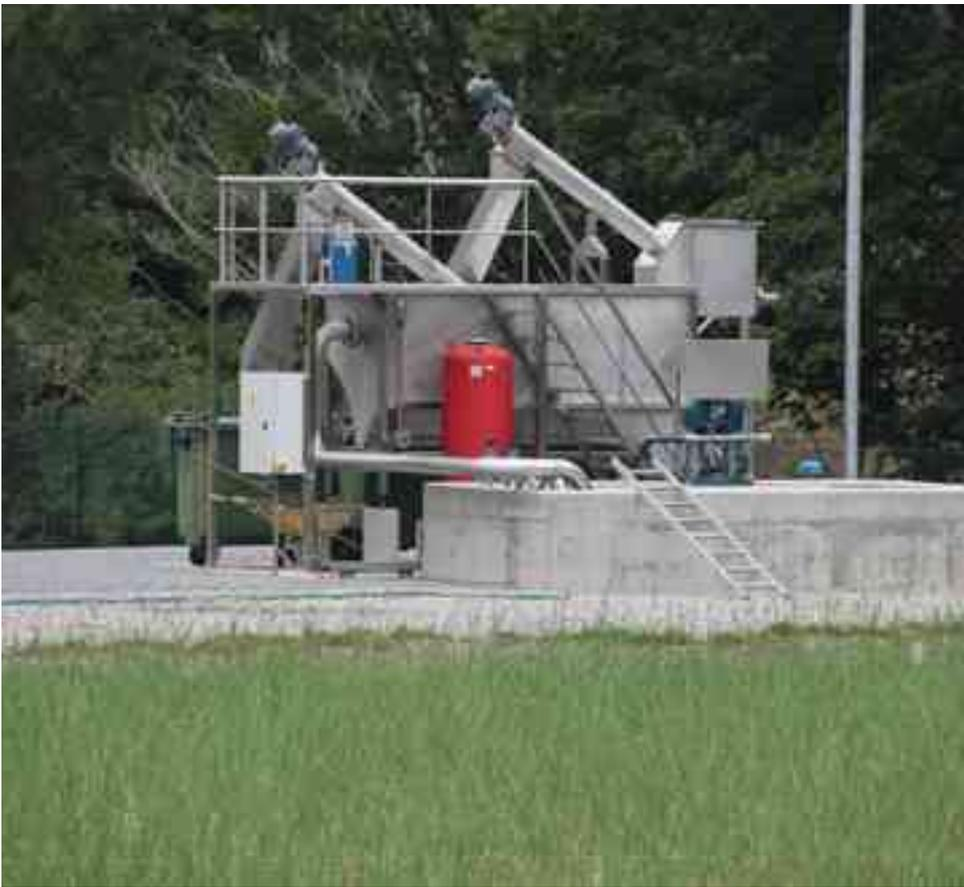
The elements in the water line are one header pumping set before the pre-treatment consisting of a compact unit where solids to be filtered, grit and grease are separated followed by a recirculation catch pit and homogenising of the influent before its entry to the pool with the macrophytes filter.
