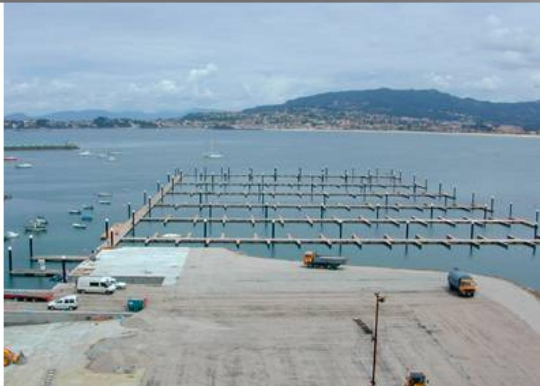
The comb-shaped layout of pontoons provides 297 moorings. The outer face of the casting pontoon and that of pontoon number 7 are used as reception and for vessels in transit, thus providing a total of 319 moorings. The pontoons are formed by an ASG T6 state aluminium structure with rot-proof tropical wood paving and floats of polyester reinforced with glass fibre. The minimum width for the interior ones is 2.50 and for the outer ones, 3.0 m, reinforced.
