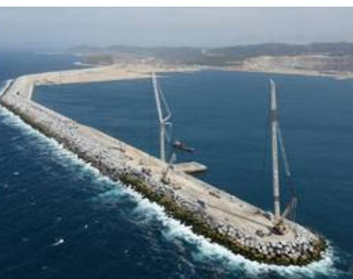
A transverse mole of precast concrete caissons (51.10 x 20.50 m) with a depth varying from 21 to 27 m long. An edge beam 5.35 m deep is located on the caissons to support the outer rail of the crane, the mooring bollards and the fenders. The crane's inner track is 18 m from the outer one on a 1 m beam with a concrete slab 45 cm thick between the two rails.
