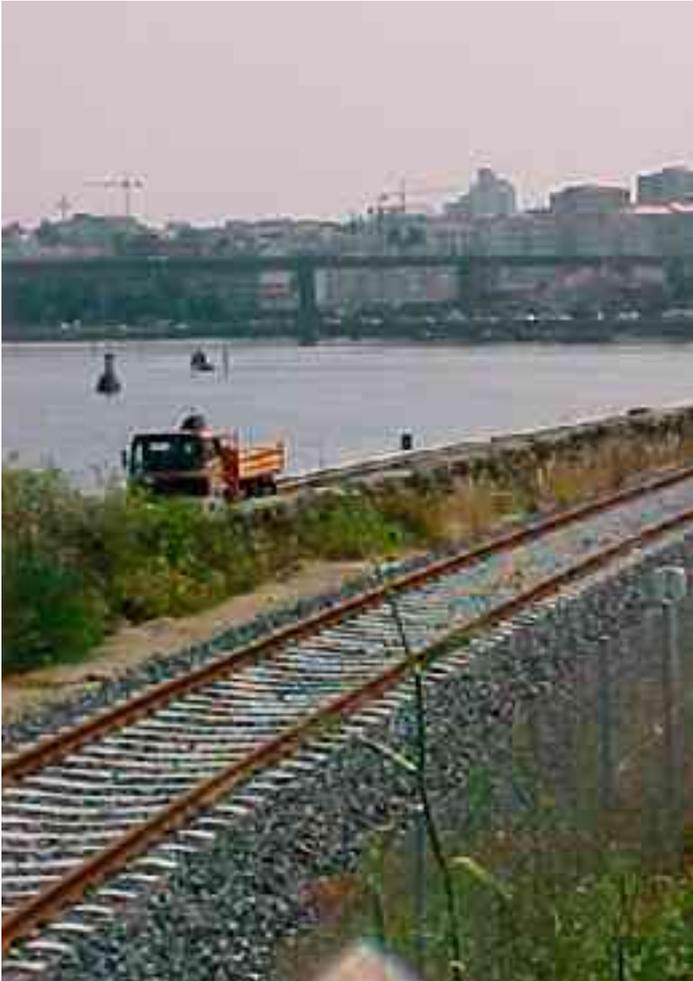
The length of the constructed track is 2,070 m. The horizontal alignment considers minimum radii of 180 and 250 m. The maximum incline was 2 thousandths on sidings and loading-unloading tracks.
