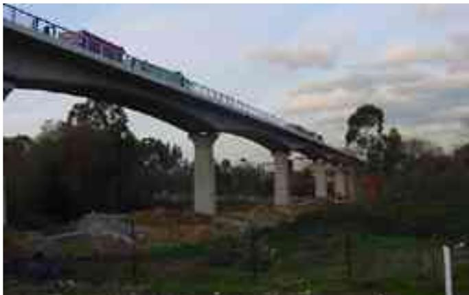
The viaduct consists of a post-tensioned lightened slab of varying thickness, arranged in 12 spans of differing lengths, totalling 412 m between the abutments. The foundations for the 11 supporting piers, which also vary in thickness and are topped with column caps to support the special-morphology deck, consist of surface shoes at the ends of the viaduct and pile caps on those nearest to the river Freixeiro, owing to the height of the water table in that area.
