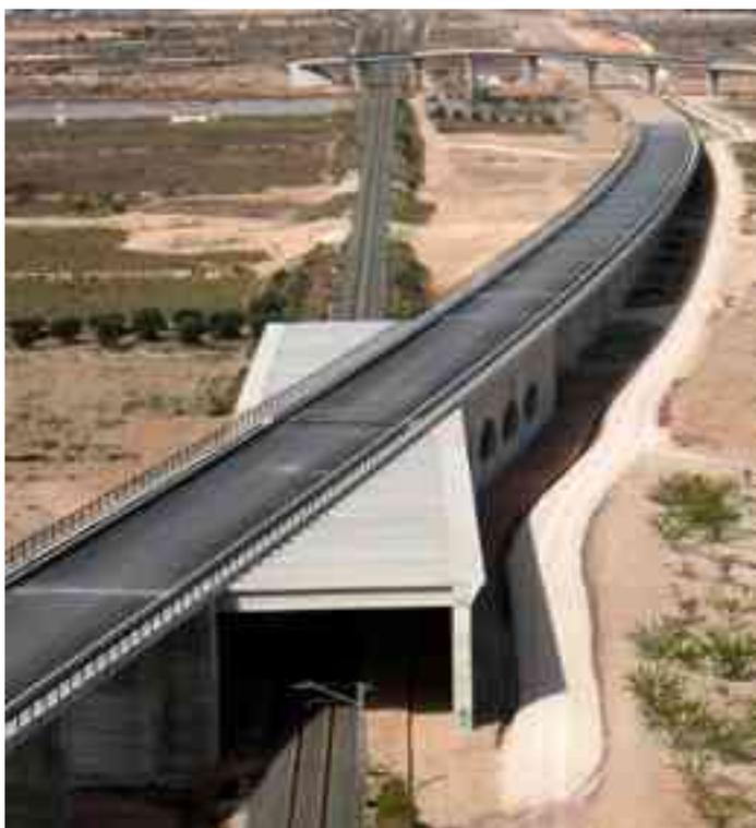
The project also includes the construction of a 1,231 m tunnel - 890 m centre section underground, 216 m entrance and 125 m exit (artificial tunnel).
