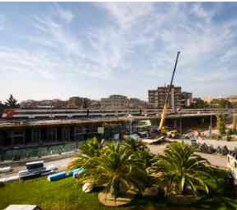
The project consists of replacing an embankment with a viaduct to eliminate the barrier effect of the embankment. The embankment impedes the transverse permeability of an urban area of Cornellà. The viaduct allows the road system to be integrated into the urban landscape.
