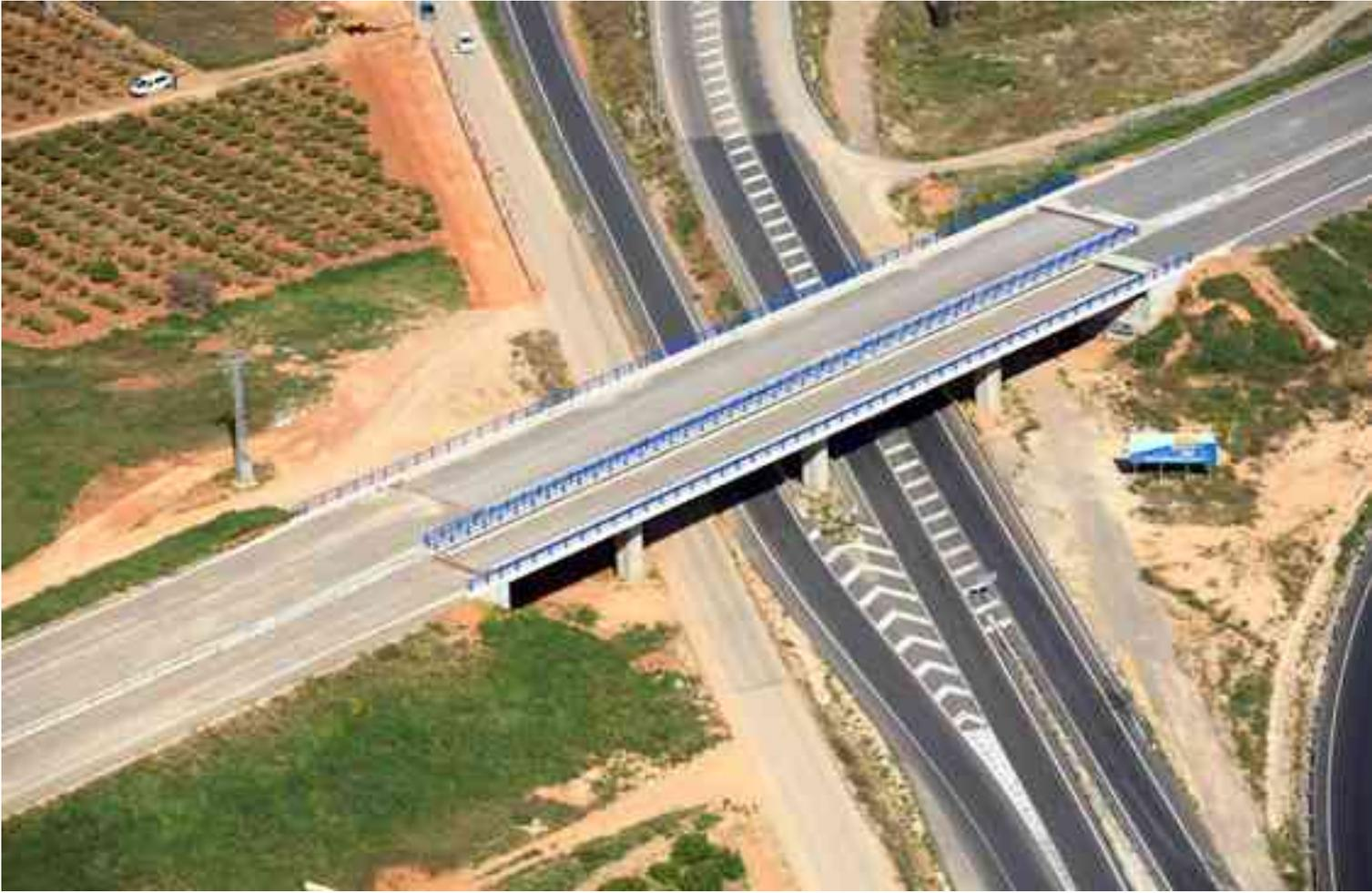
In relation to the structures, 12 viaducts were built, measuring between 45 and 141.50 m long, as well as 4 overhead passes built of reinforced or post-stressed concrete or prefabricated beams, and 8 underpasses. The construction of these structures involved the manufacture of 4,127 linear m of piles with a 1.8 m diameter, 3,359 piles with a 1.5 m diameter and the employment of 8,000 tonnes of reinforcement steel bars.
