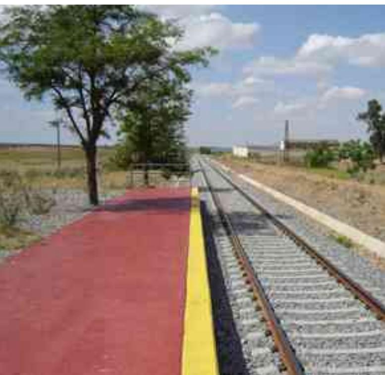
The track layout will be regularized, adapting it to speeds that are compatible with the existing infrastructure and the entire track is to be replaced with UIC-54 rail, PR-01 multi-purpose monobloc sleeper, type "2" siliceous ballast with 30 cm under the sleeper and 15 cm at the Villanueva de la Serena and Don Benito stations, and type C weldable deviations.
