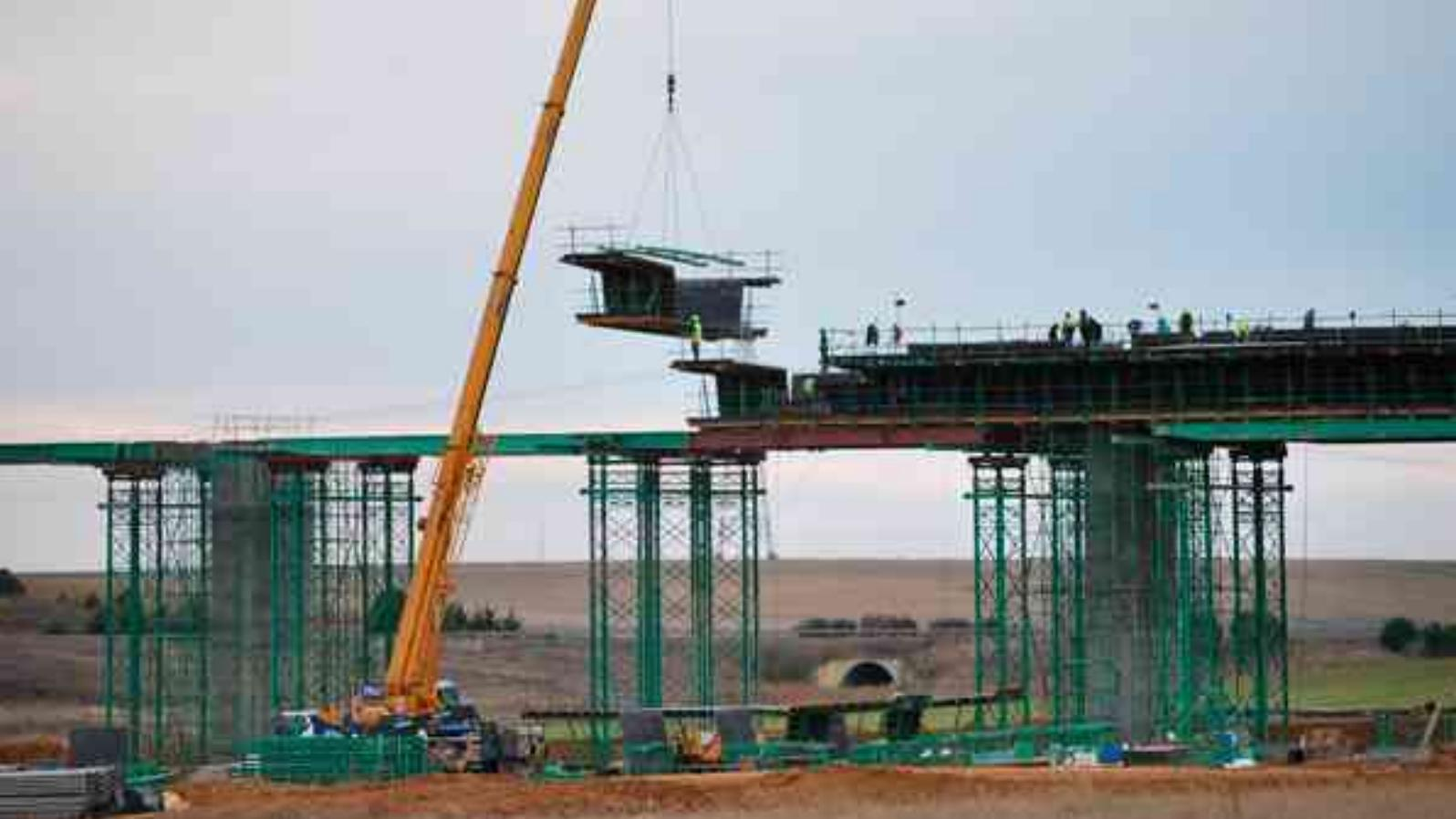
The work will fundamentally be carried out on embankments, with the majority of the materials being loaned. In terms of structures, there basically are three viaducts, Granja, Utielga and Olmo. All of them have a hyperstatic structure of reinforced, post-tensioned concrete made up of continuous box girders constructed using centering, with supports founded on piles.
