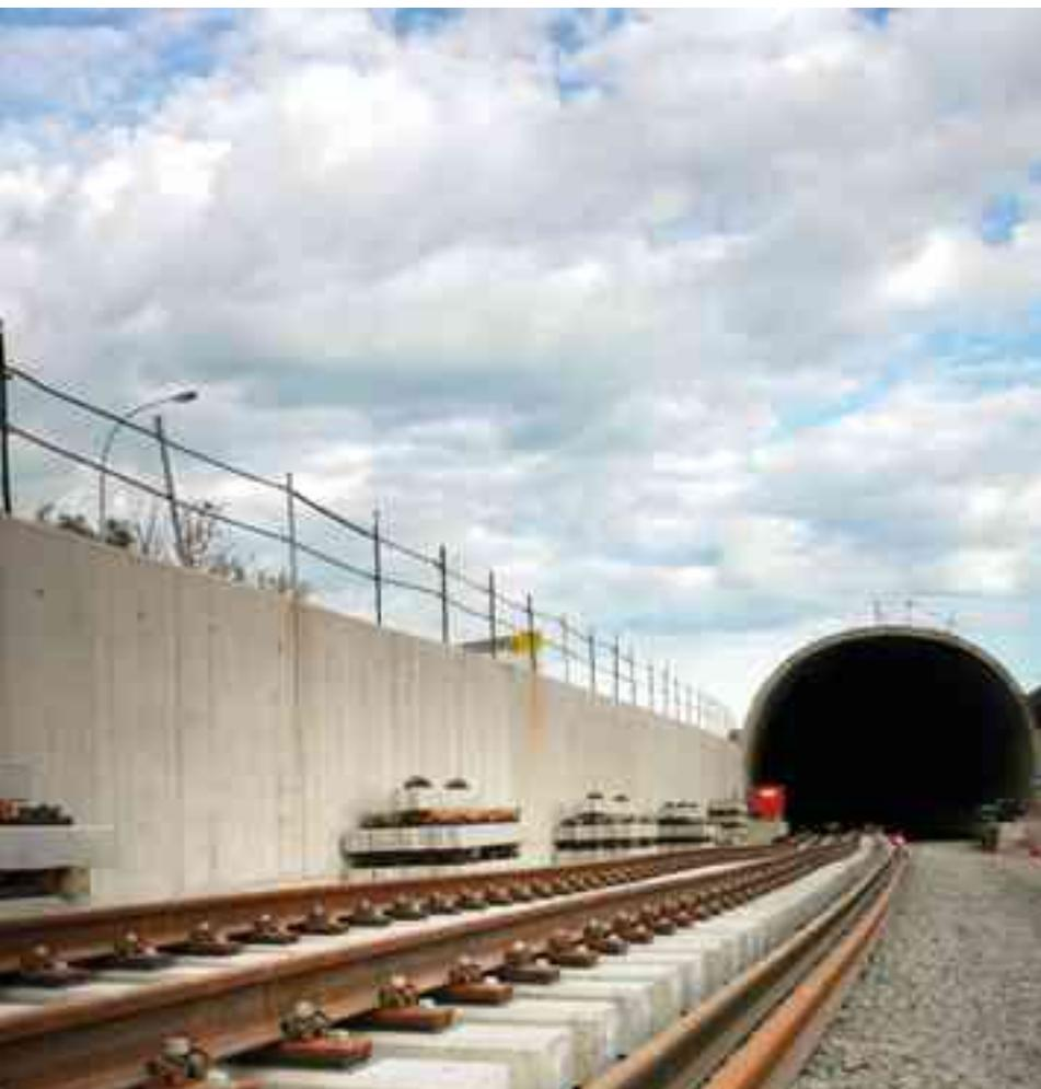
The planned track mounting system is on ballast, with the exception of the La Cabrera, Buñol and Torrent tunnels and the viaduct over the river Turia and the artificial tunnel at the entrance to Valencia, where the track shall be mounted on concrete slabs totalling 31,500 m of track on slabs. In addition within these works the laying of track for the Almussafes – Valencia commercial line will be carried out with multipurpose sleepers and Iberian width.
