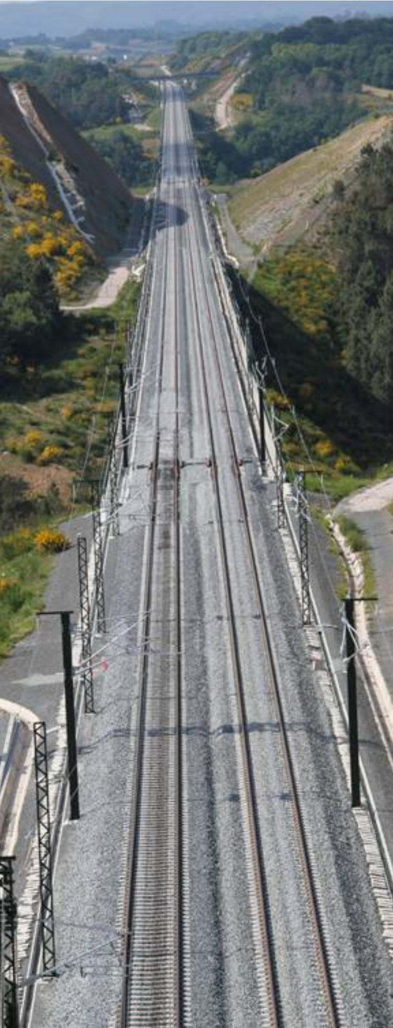
The project corresponds to the O Irixo – Santiago section, which is 59.25 km long and in which polyvalent concrete sleepers and UIC60 track are assembled on Iberian gauge.
