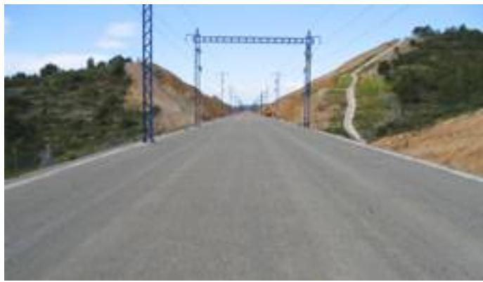
The works carried out consisted of the supply of 318,299.20 m<sup>3</sup> of type A siliceous ballast and the layout of a 54.9 km section of High Speed track between the districts of Alcover (Tarragona) and Vilafranca del Penedés (Barcelona), of which 49.1 km have a double track yard and 5.8 km have two single track yards, with a total of 109,736 m of track.
