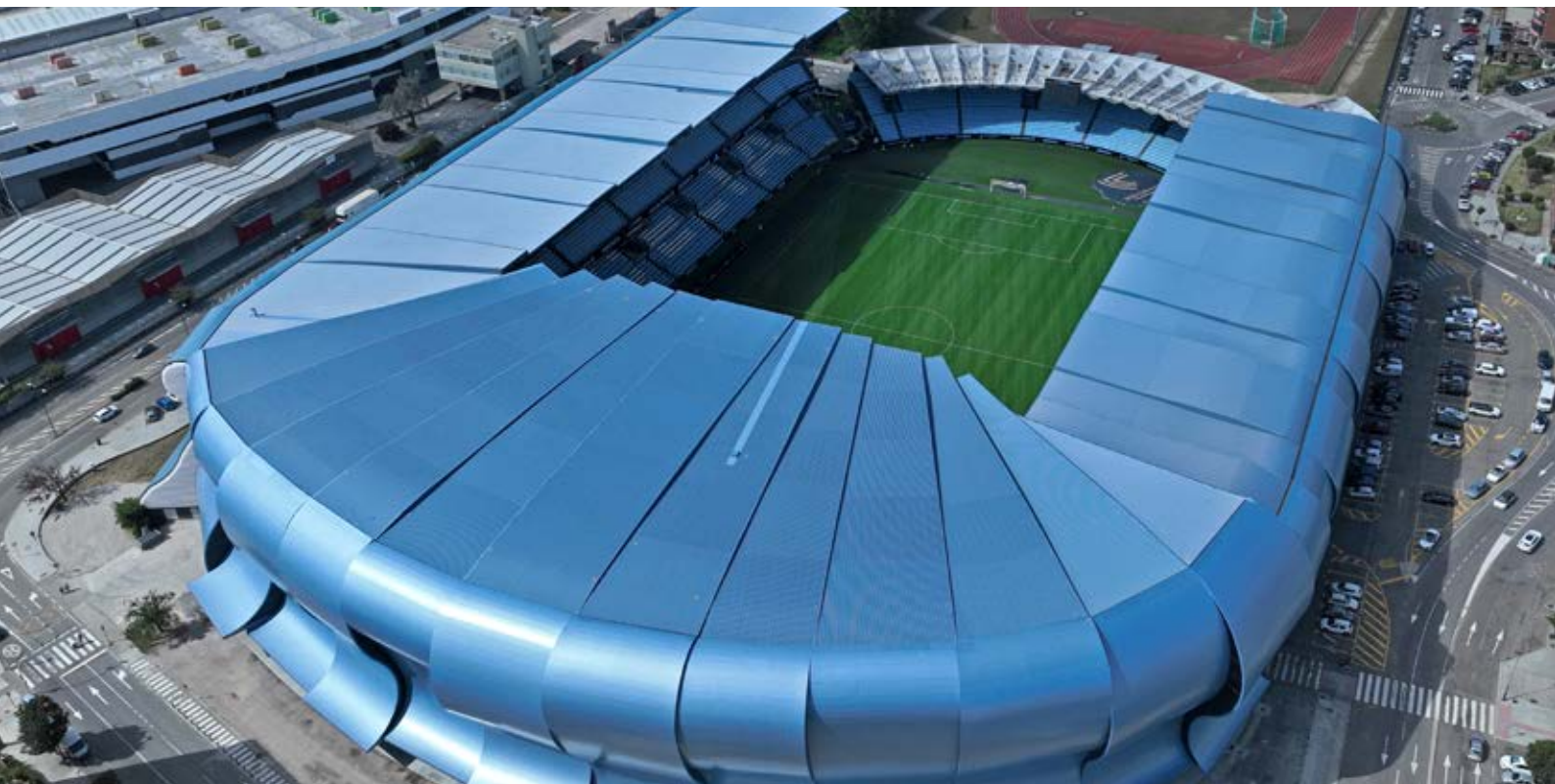
Reforma Estadio Balaidos en Vigo, España | Balaidos Stadium renovation in Vigo, Spain
